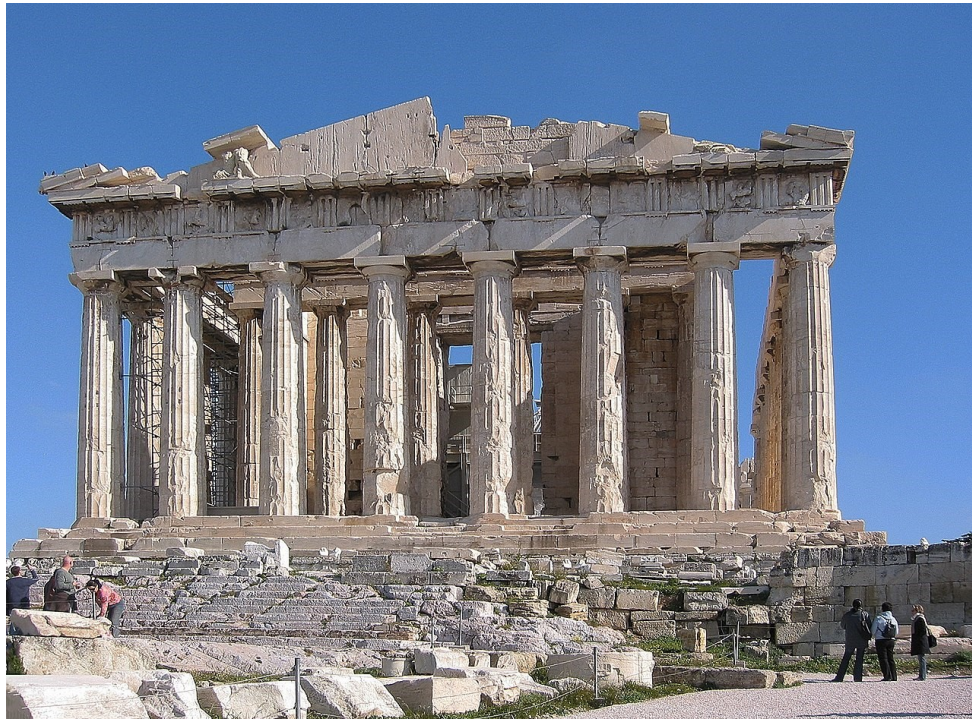
Contemporary view of the Parthenon.
