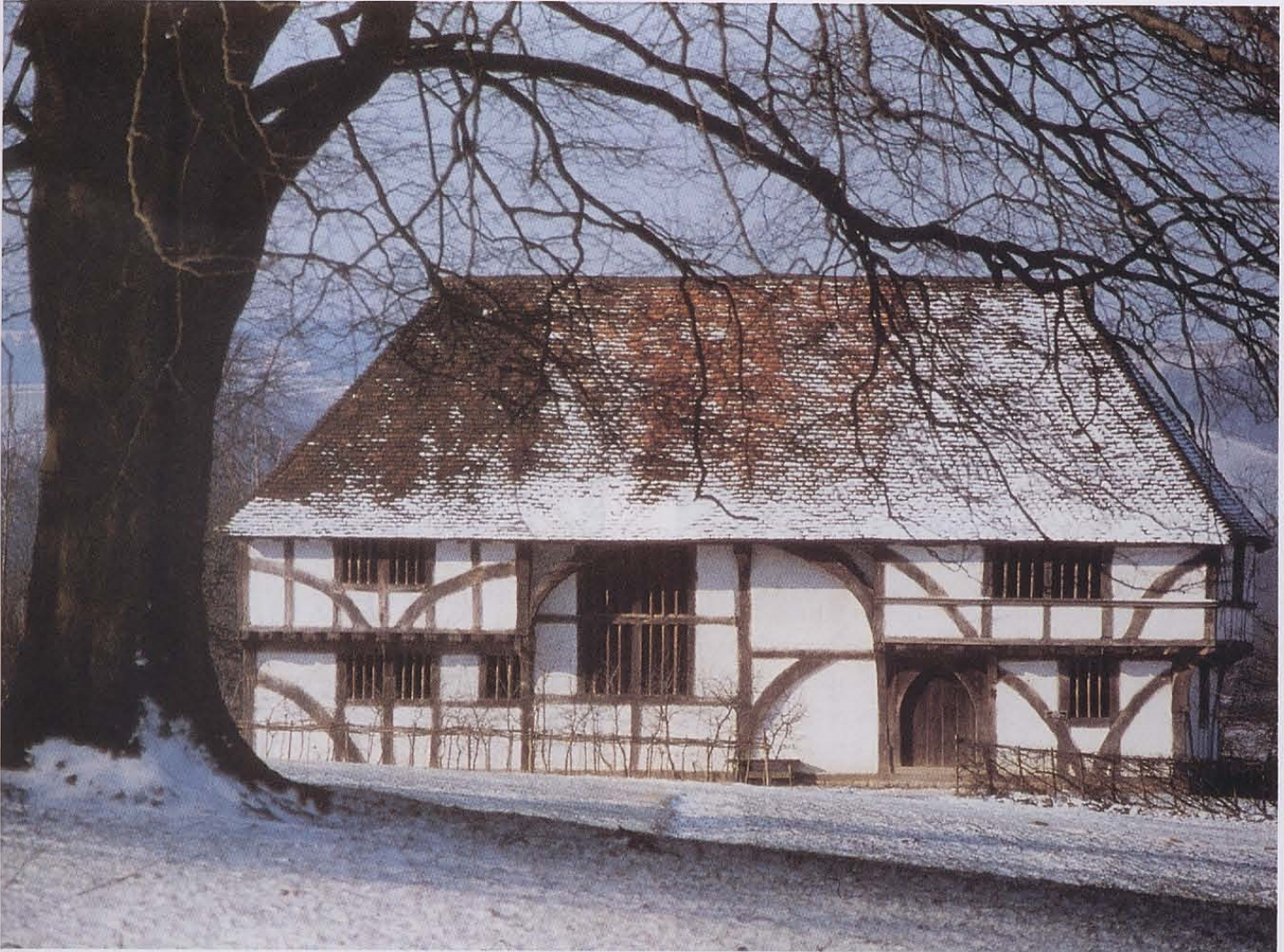
Bay Leaf Farm, a fifteenth-century Kent farmhouse, a timber-frame building with walls made of "wattle and daub", basically sticks and mud. This was a very effective type of building, but required skilled carpenters to make a strong frame. One man who did not like this new method called these houses little more than "paper work". But examples are still lived in as ordinary homes in many parts of England.
